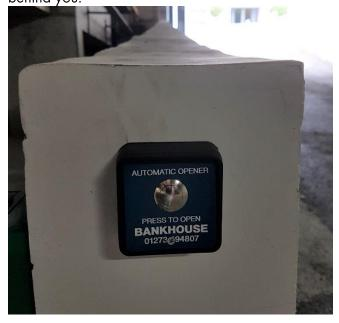
As the ramp is one of the fire escape exits from the underground car park there is a manual override button located at the bottom of the ramp. If you press this button the gates will open to let you out. You can also use this button to exit via the ramp on foot. The gates will automatically close behind you.
